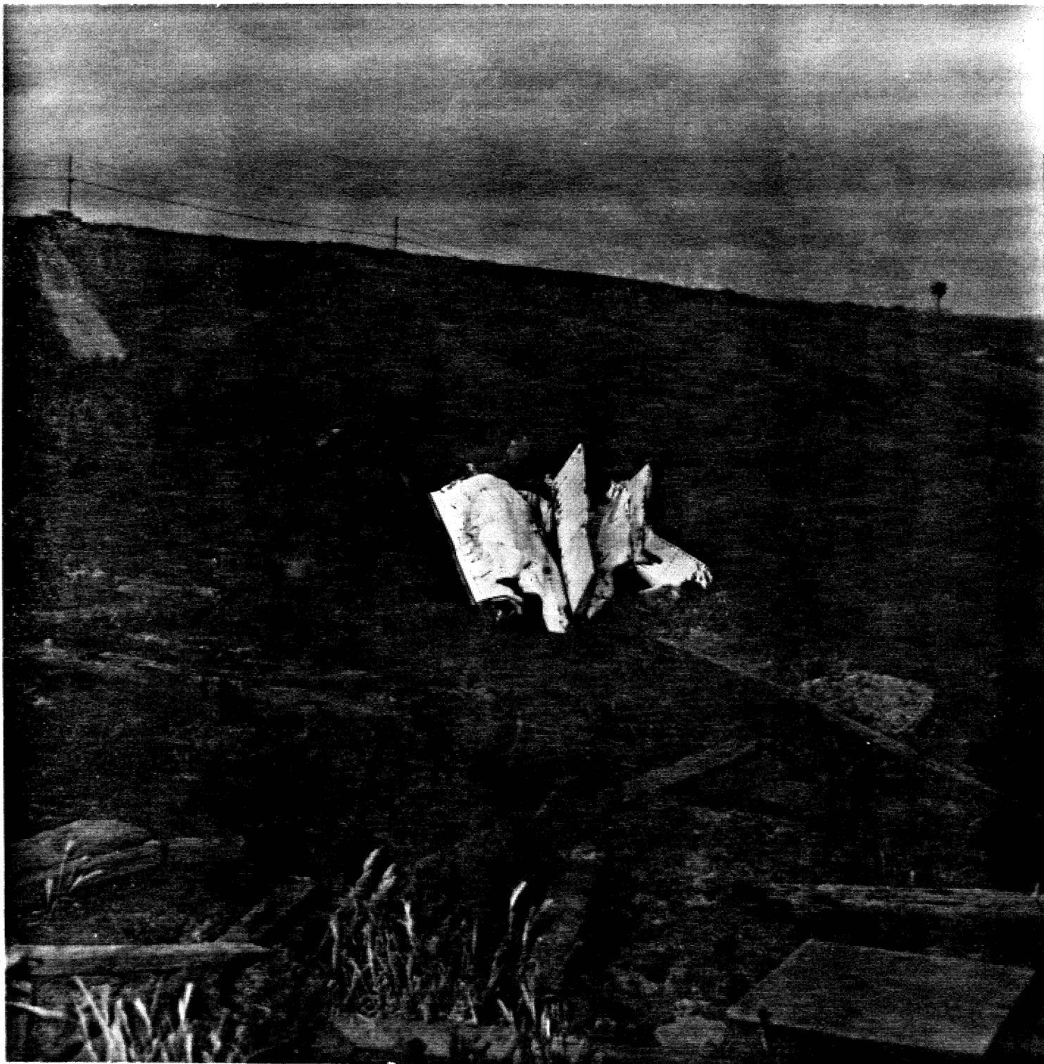
19. Piece of left outboard wing skin with aileron.
